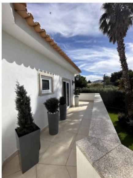
Fig. 6.1a — Veranda with the roof eave above; no gutter, and the open section takes the run-off.
